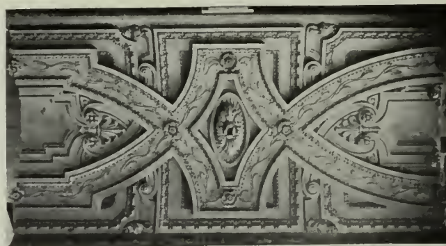
CEILING PANEL IN MAIN LOGGIA, STATE EDUCATIONAL BUILDING, ALBANY, N. Y. Executed in white, cream and light blue terra cotta by Atlantic Terra Cotta Company. Palmer & Hornbostel, Architects.
